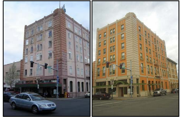
The Temple Hotel before façade restoration, left, and the St. George Plaza after façade restoration, right.
