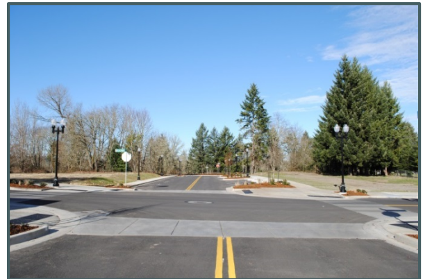
After: Public Improvements Installed (2010)
