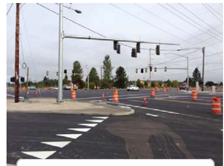
Aumsville Highway Signal Improvement
