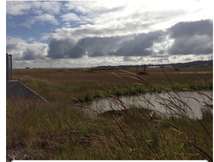
Constructed Weir and Wetlands
