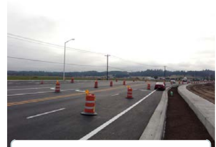
Aumsville Highway Widening
